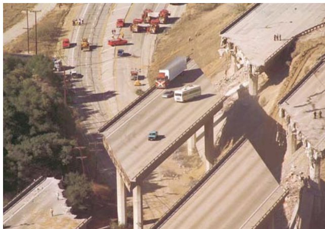
Fig. 3. Example of bridge collapse after an earthquake
